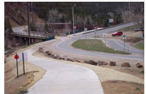
The new bridge and intersection on the Clear Creek County Greenway.
