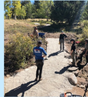
MRHI Stewardship Crew improved tread with crush fill and compacting at Puma Point!
